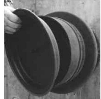
4. Place second end cap on sleeve. Check to determine that the cap is properly inserted.
